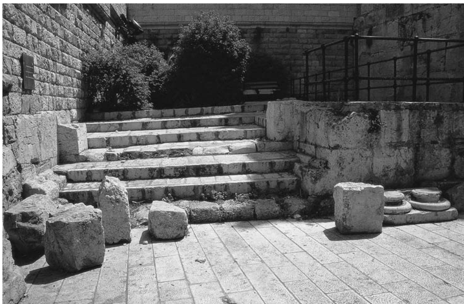
Plate 7.5 Remains of the Crusader barbican outside St Stephen's Gate (photograph by Gabi Laron).
